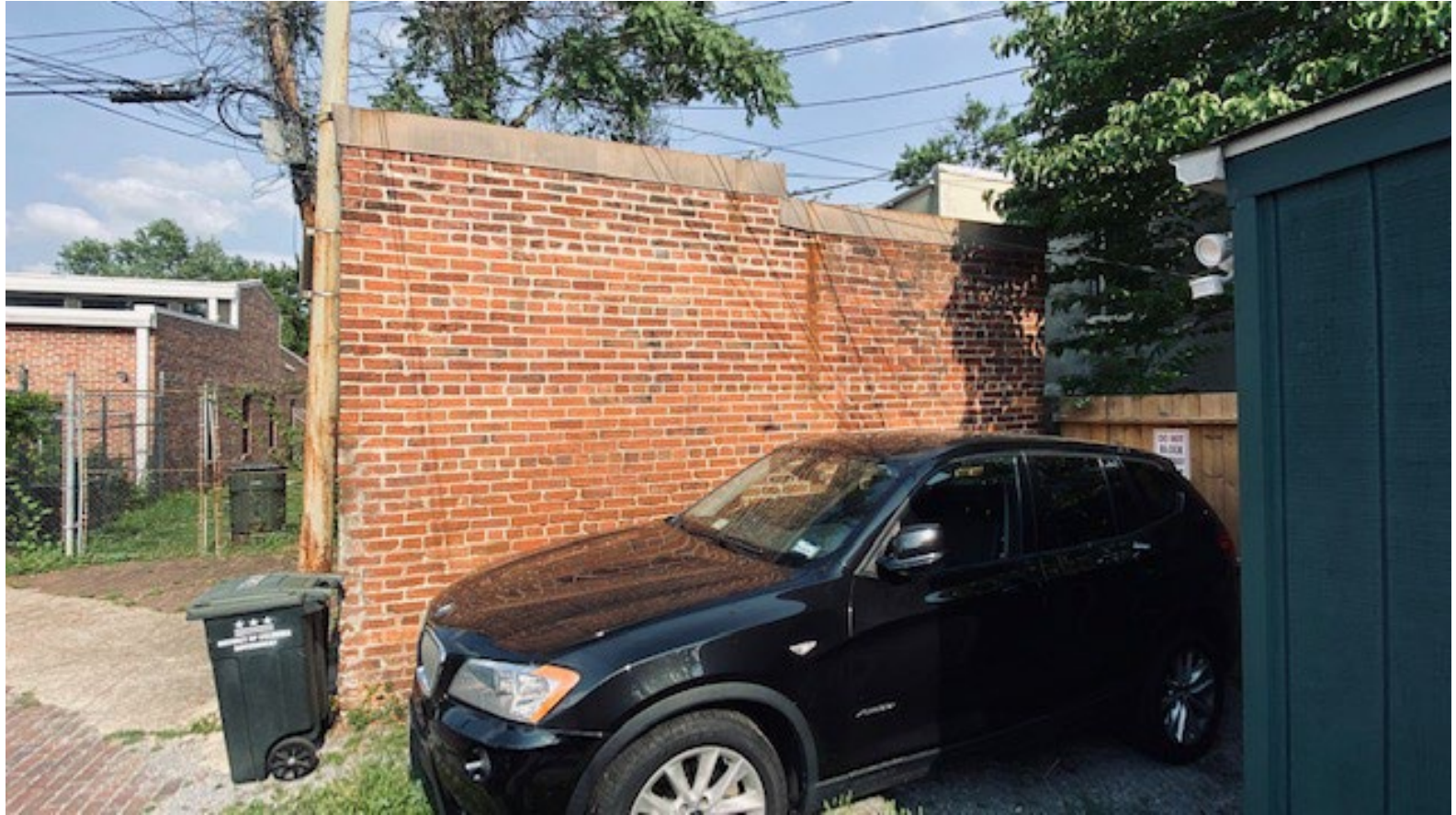
Side View from Adjacent Parking Pad
